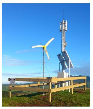
Web Access Waikato and Wanna Internet have also identified the aerial type that will be installed in Ngaruawahia. The installation typically comprises a steel pole of no more than 7m in height with solar panels and an equipment cabinet bolted to it. The design has been installed on many hilltop sites and has been found to be non-intrusive and due to its small size does not require Council consent.
